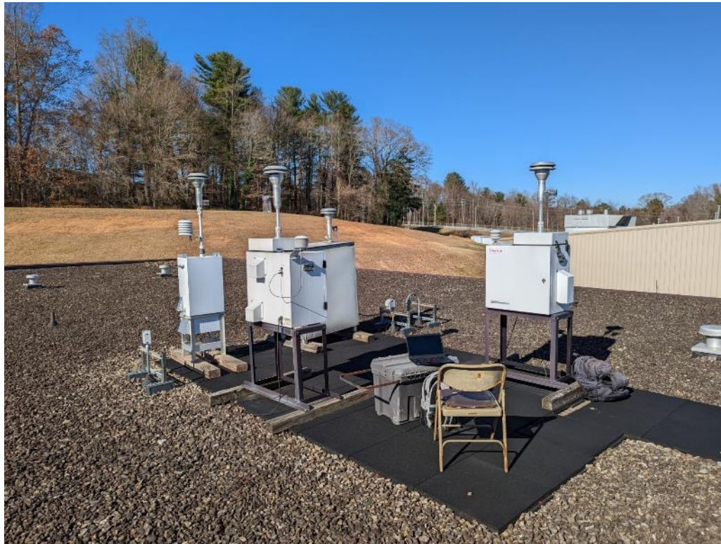
Existing roof top site
