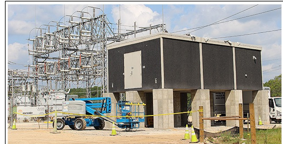
Entergy Corp. elevated a substation in Texas that was damaged during Hurricane Harvey. Entergy
