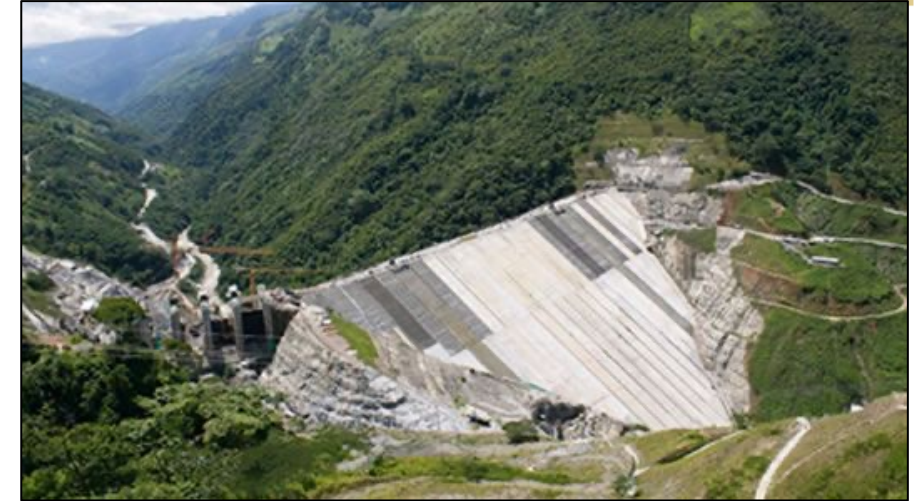
Colombia's US $4bn Ituango hydroelectric project was hit by two significant landslides in 2018. Source: bnamericas, May 28, 2018.
