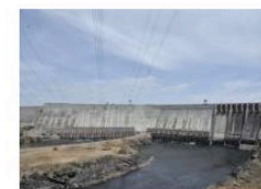
Following rains, the water level of the Guri Dam has increased by 13 centimeters in two days (Fae photo)
